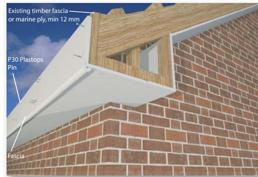
Fig. 17. Standard over-fascia installation.
