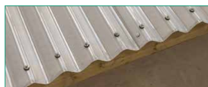
1 Primary Fixing At every corrugation
